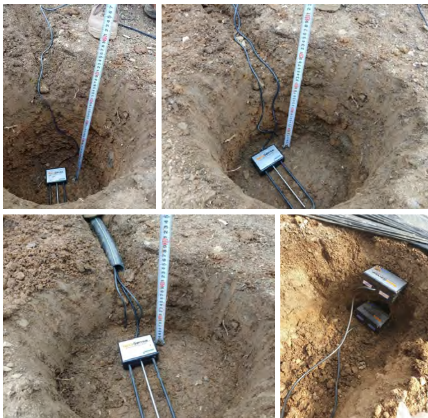
Figure 5. Sequential installation of three Netasense soil moisture sensors in the excavated pit on the top of each other and two sensors in the side wall of the excavation (bottom right)
